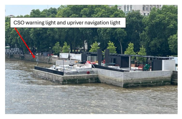
The lights will flash a yellow alternating 1 second pattern, visible day and night at a range of up to 200m, whenever the CSO is discharging or likely to discharge.
