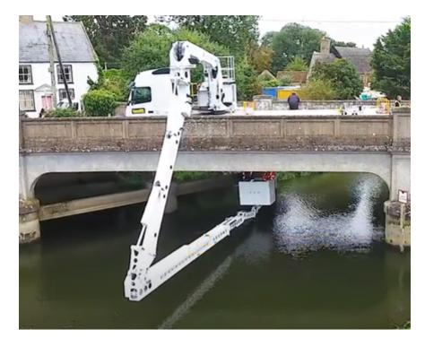
Works will be conducted from the road bridge using a bridge access platform, similar to that shown above, and a mobile crane. The maximum boom radius of the access platform is approximately 19m from the bridge. No vessel should enter the area shown on the chart other than those involved with the works.
